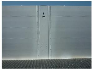
Side panels: Check that the rivets are tight
