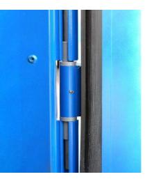
Check hinges for damages and correct operability Check hinge mount for damage and tight fit
