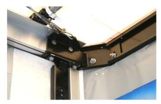
Front cover: Check that the screws are tight, check wire link (cover and wire stiffening)
