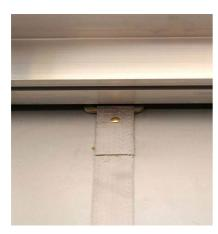
Sheaves: Check that rivets are tight, Check straps of damages and cracks
