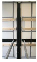
Central posts: Check that all rivets are screws are tight
