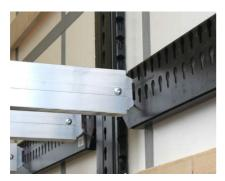
Girders: Check for proper state, check that rivets are tight
