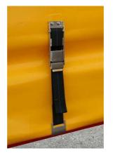
Flat hooks: Check that rivets are tight and the strap is undamaged
