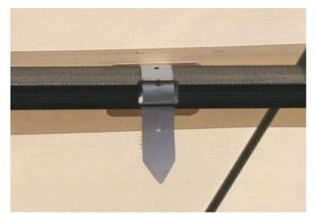
Check tensioning strap for damage
