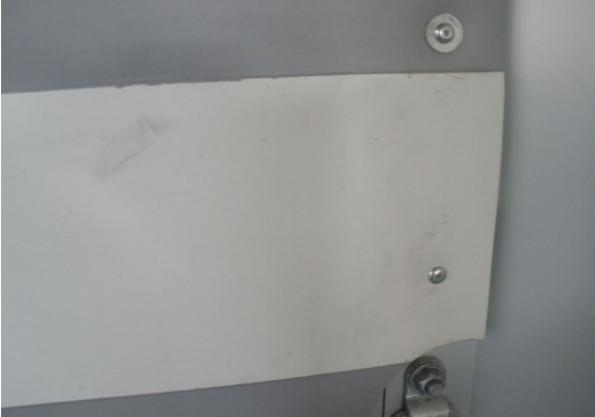
Inner and outer GRP sandwich panels: Check that all rivets and screws are tight; general inspection of sandwich panel
