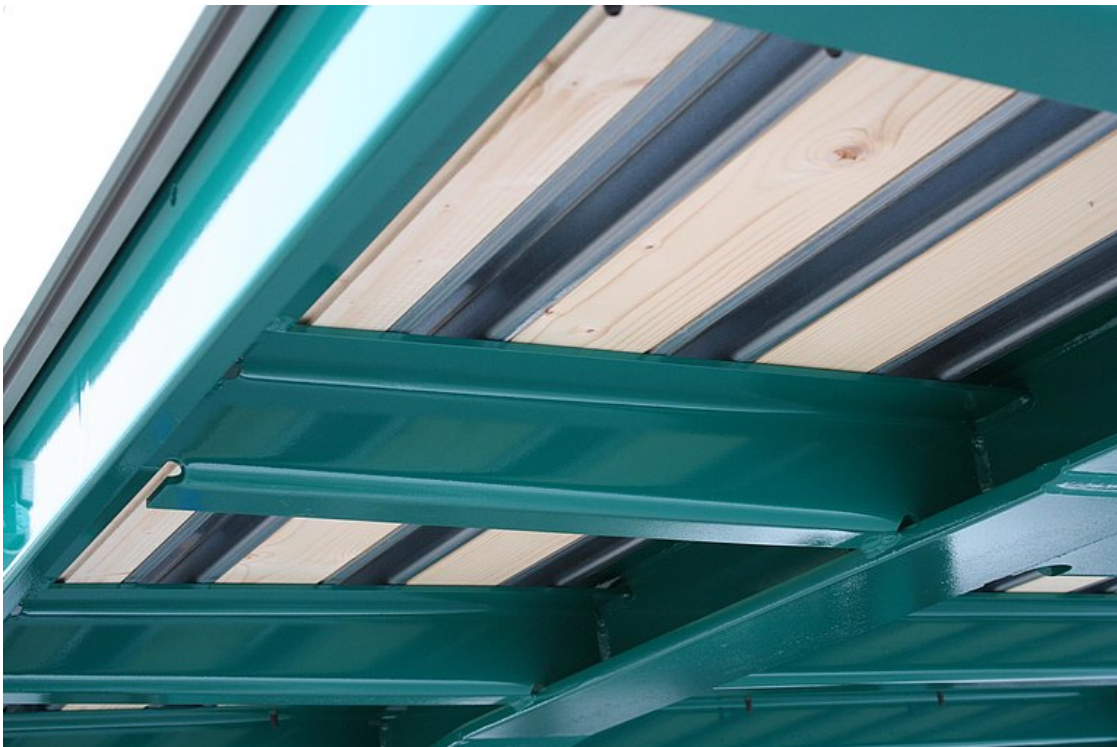
Double floor consisting of subfloor with integrated steel omega profiles beneath resin-coated wear floor
