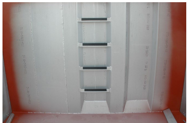
Interior: Check the weld seams for cracks
