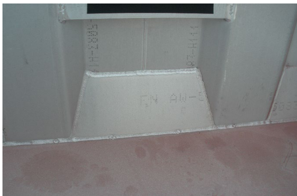
Interior reinforcement: Check the weld seams for cracks
